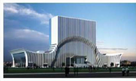
Xinjiang Weital Building
